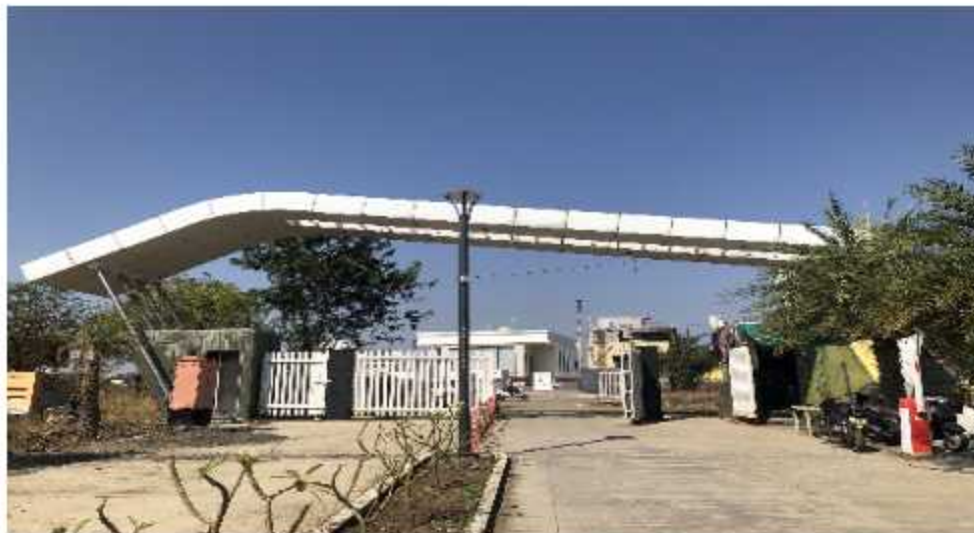
Compound wall With Concertina Fencing
